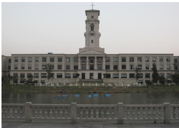
Administration Building, University of Nottingham, Ningbo Campus, China
